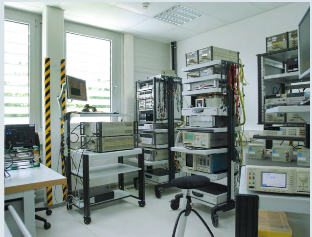
High-quality references at the electrical primary laboratory
